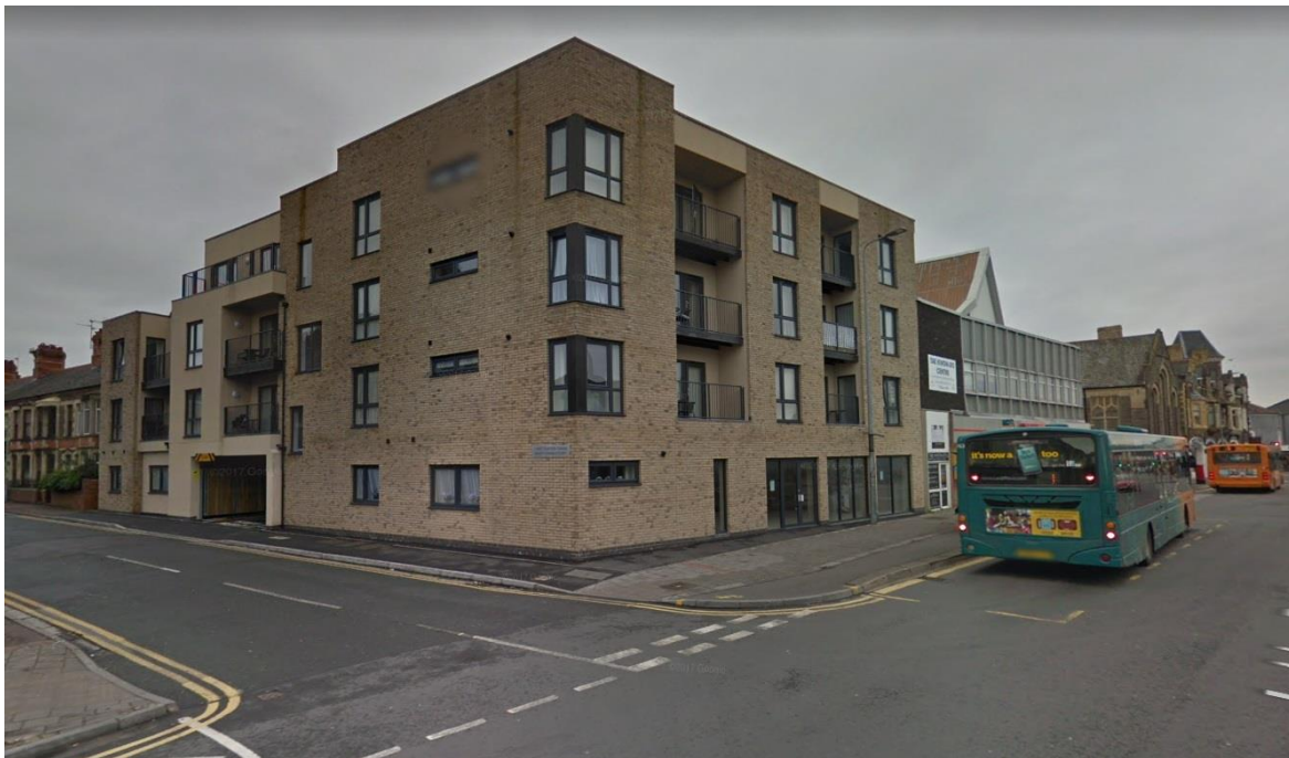
Social housing on previous Canton police office building with balcony amenity space
